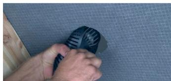
3 Holding firmly onto the fixing strip, squeeze the grill section of the KimaAir Outside-In and push through the hole
